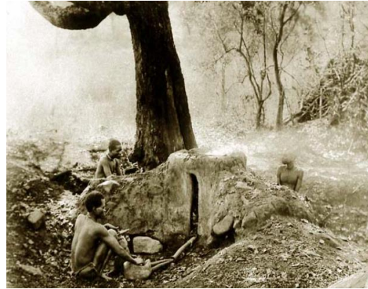
Venda-type iron smelting furnace from 1888
